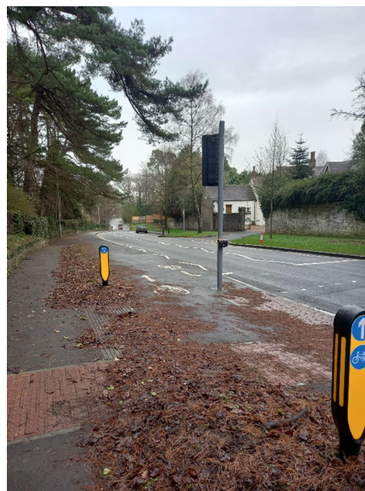
East Bound controlled crossing at Clyne Drive
