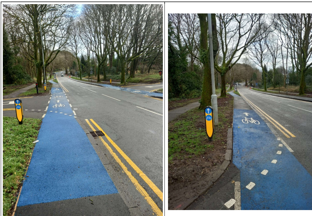
Southdown Avenue junction with Mayals Road - Westbound
